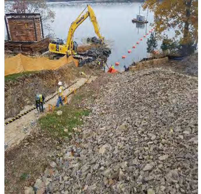
Fig 8: Pulling cable at Getchell property/west side of the Bay. Viewing east. (10-25-19).
