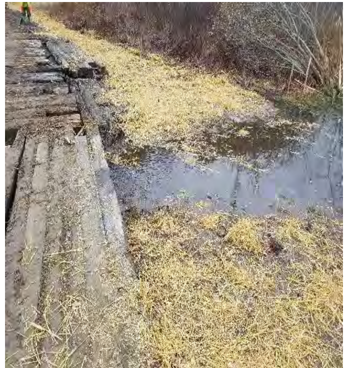
Fig 24: Knights Brook flowing after by pass removal at Frink farm. Viewing east. (10-29-19).
