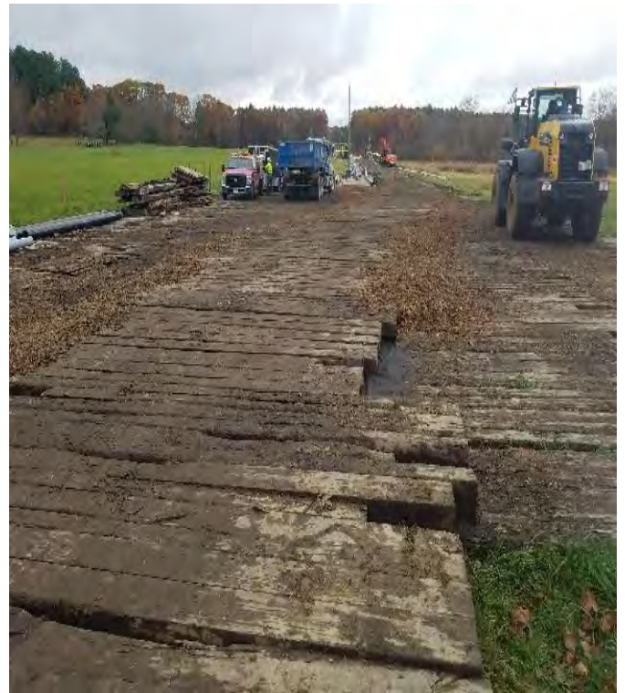
Fig 29: Additional mats and stump grindings added to access road at Frink farm. Viewing east. (10-30-19).
