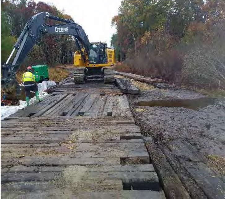
Fig 13: Beginning to remove stream bypass in Knight's Brook tributary. Viewing west. (10-28-19).
