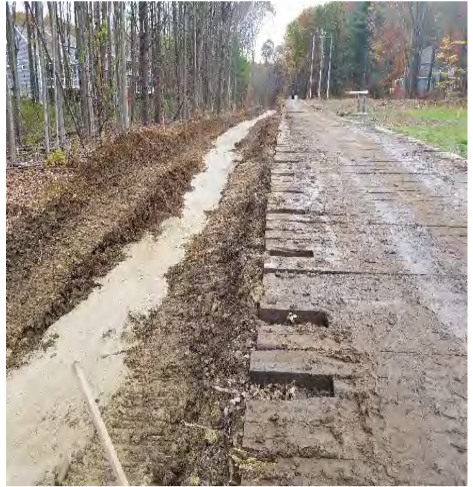
Fig 26: Float fill poured in trench between Str. 107 and Nimble Hill Road. (10-29-19).
