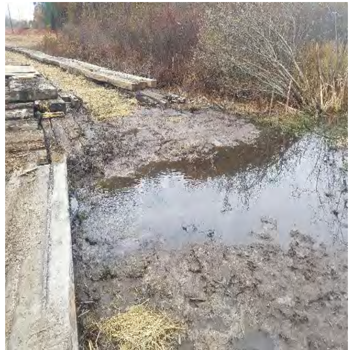
Fig. 18: Knight's Brook tributary flowing after bypass removed. Viewing east. (10-28-19).
