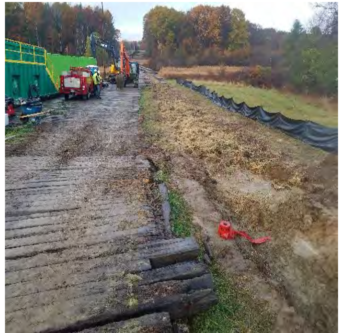
Fig 20: Restored trench area in agricultural zone at Frink farm. Viewing east. (10-29-19).
