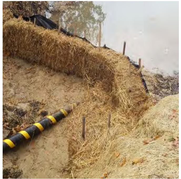
Fig 10: Sediment controls in trench at Gundalow landing/east side of the Bay. Viewing west. (10-28-19).
