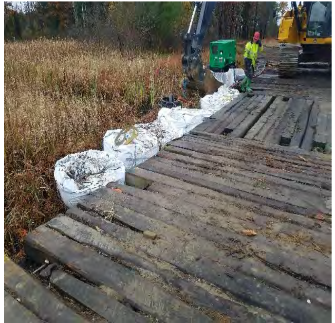
Fig 12: Beginning to remove stream bypass in Knights Brook tributary. Viewing west. (10-28-19).
