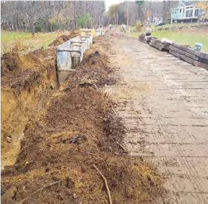
Fig 25: Trenching from Str. 107 to Nimble Hill road. Viewing west. (10-29-19).
