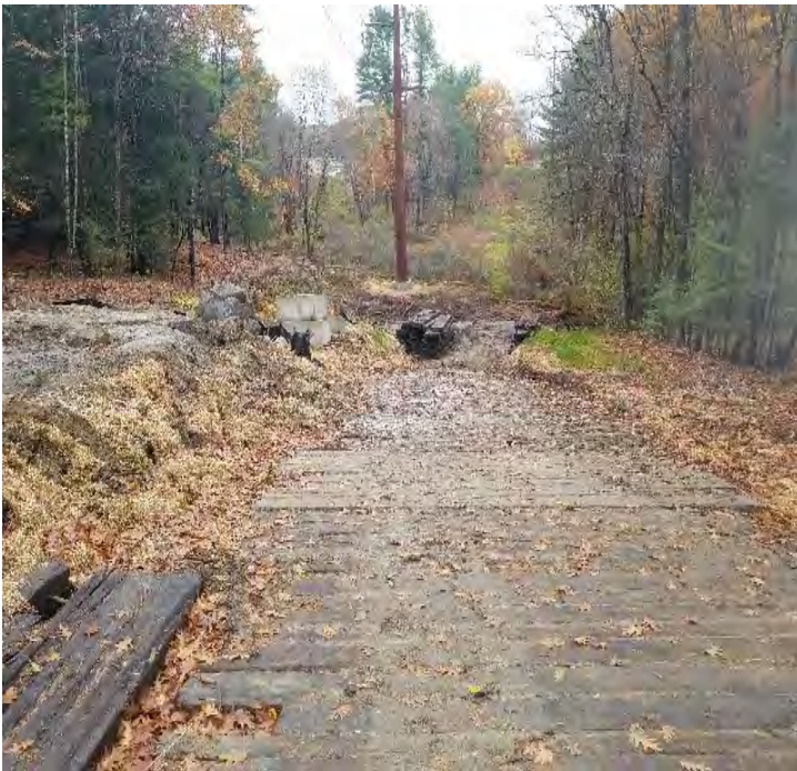
Fig 15: Timber mats are being removed around Strs. 28-29. Viewing north. (10-28-19).
