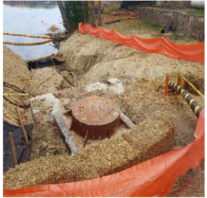
Fig 6: Vault and trench at Gundalow landing/east side of the Bay. Viewing west. (10-25-19).
